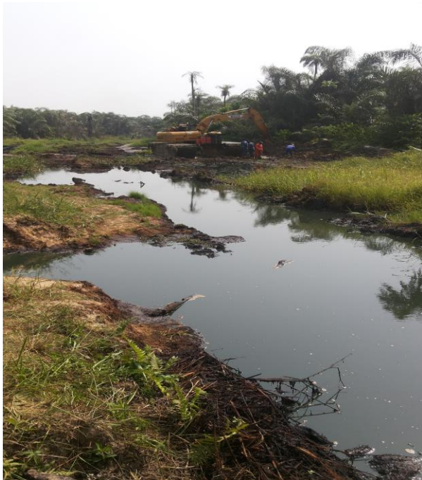
DIGGING OF NEW RETENTION PIT
