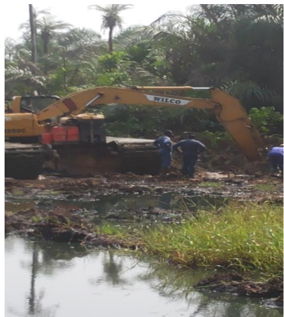
DIGGING OF RETENTION PIT
